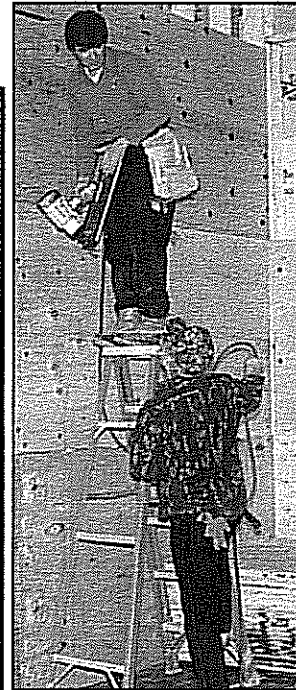
Remodeling the gym
