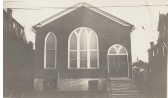
After the make over, 1930
