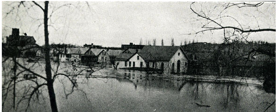
Church Building - Center
