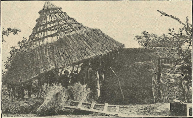
Africa—Nigeria. Putting the roof on a house.—Joseph Ummel.
