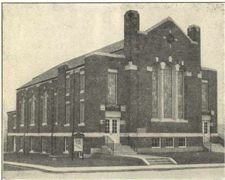
Bethel Mennonite Brethren in Christ Church, 418-20 Elm Street, Emaus, Pa., Rev. G. F. Yost, Pastor. The building is 48x96 feet, the lot 80x150 feet. The lot and building completely furnished, cost $41,500. Construction began June 13, 1932. Everything was finished as it is now by January 19, 1933 and dedicated January 22.
