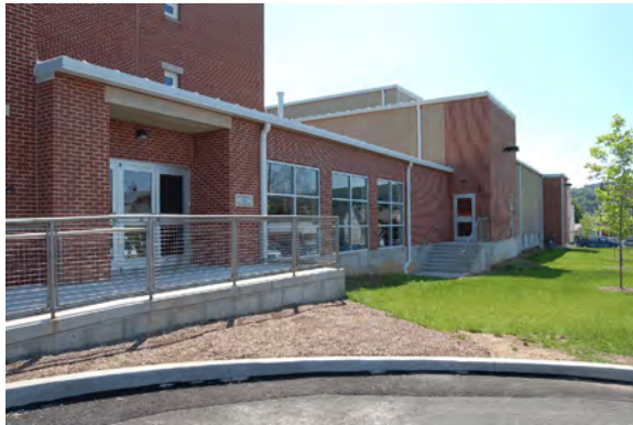
Emmaus, PA, addition - Gym, Kitchen, Classrooms
